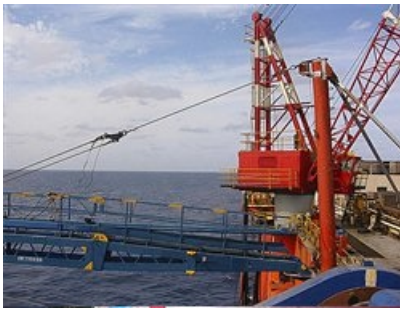
Flare Boom demounting, rerigging and installation.
