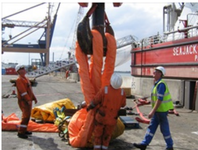
Supervision of lifting operations - OPITO level 3 riggers.
