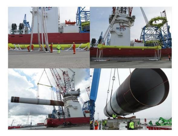
We have the expertise and experience throughout Europe of designing and creating products for bespoke lifting applications from lifting wind turbine generators to blades. Here are some photos of our custom made products in use. In the first three images you can see a wind turbines monopile being lifted with Extreema soft slings and a bespoke beam.
